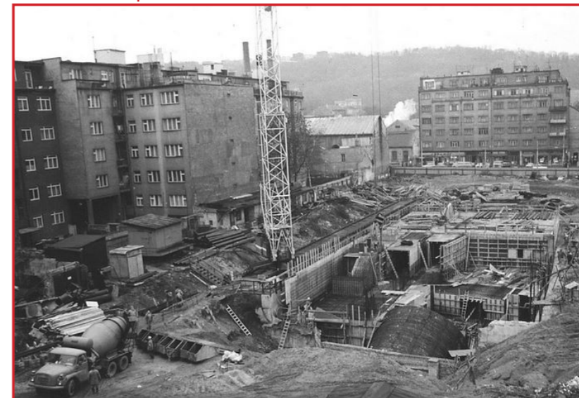
Construction of the Andel metro station - 1980's
